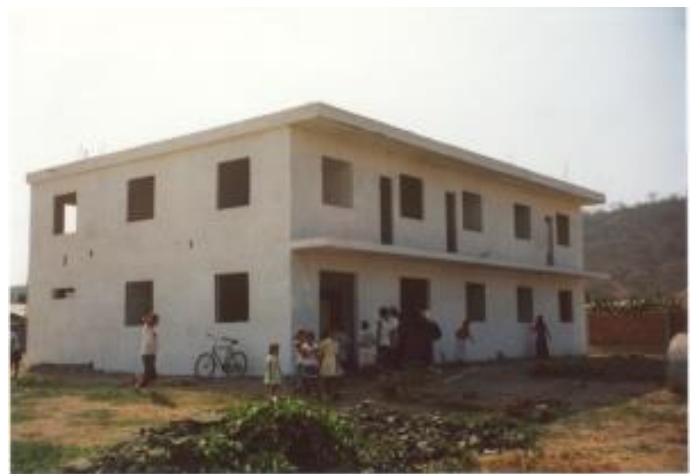
Clinic building takes on a new face
