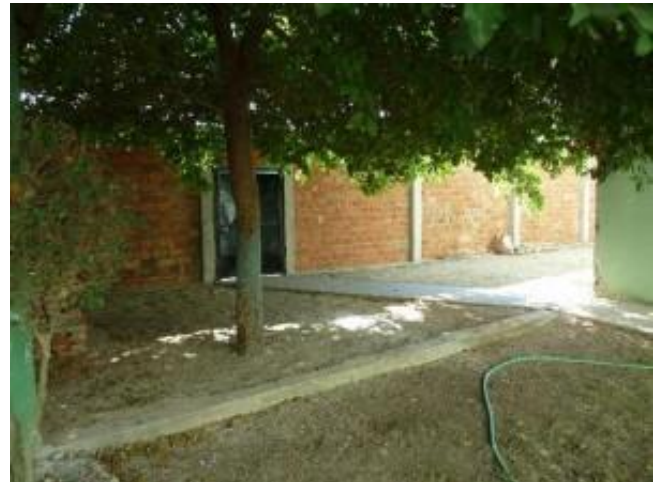
Back wall #1 completed
