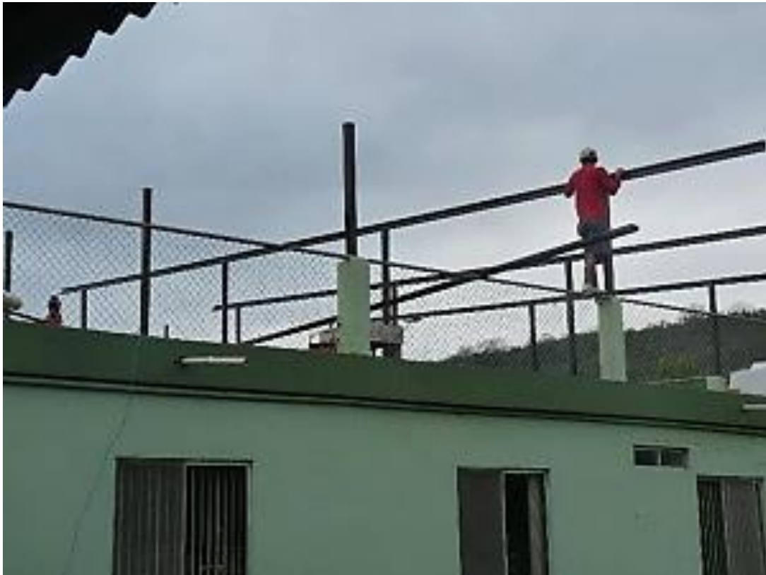
A new metal roof-our answer to the standing water problem
