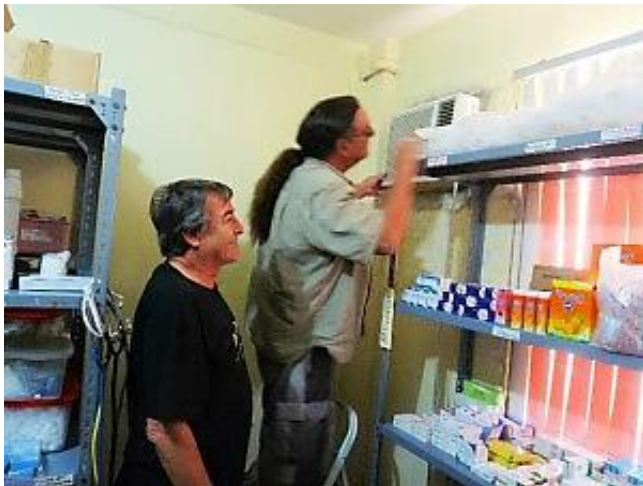
Cleaning the pharmacy's air conditioner
