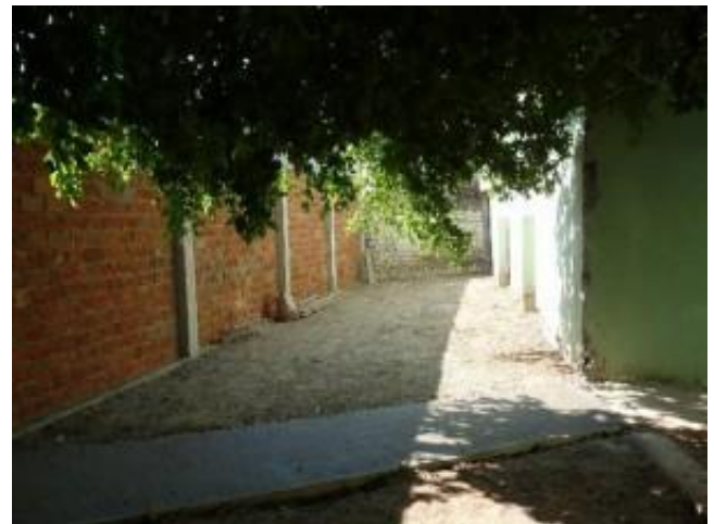
Back wall #2 completed
