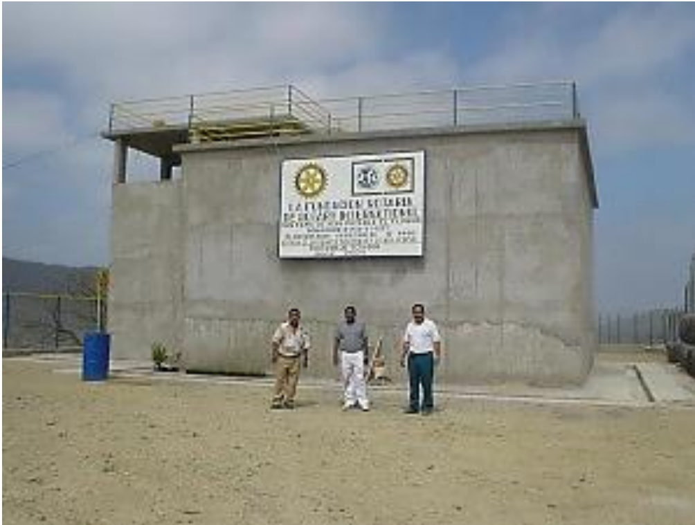
New El Floron water tank system-however the water was not potable.
